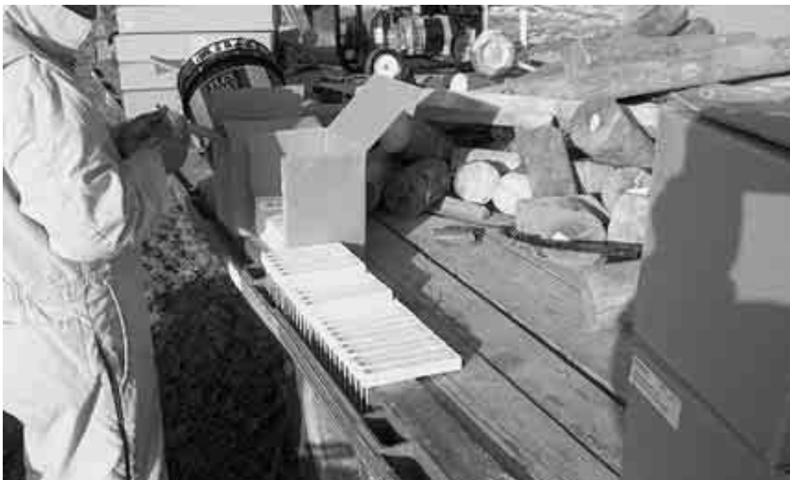
Photo 5-3. A person preparing the brackets to be nailed.
