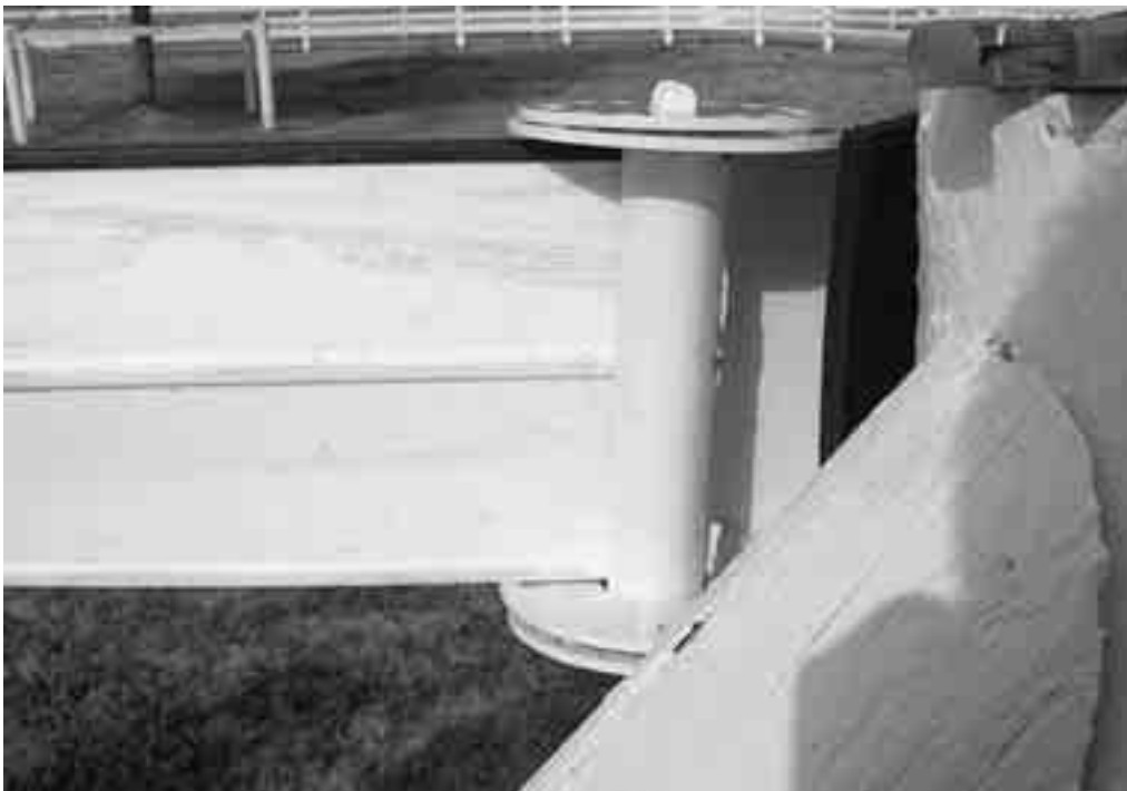
Photo A.5 Rail slid into slot of tensioner.
