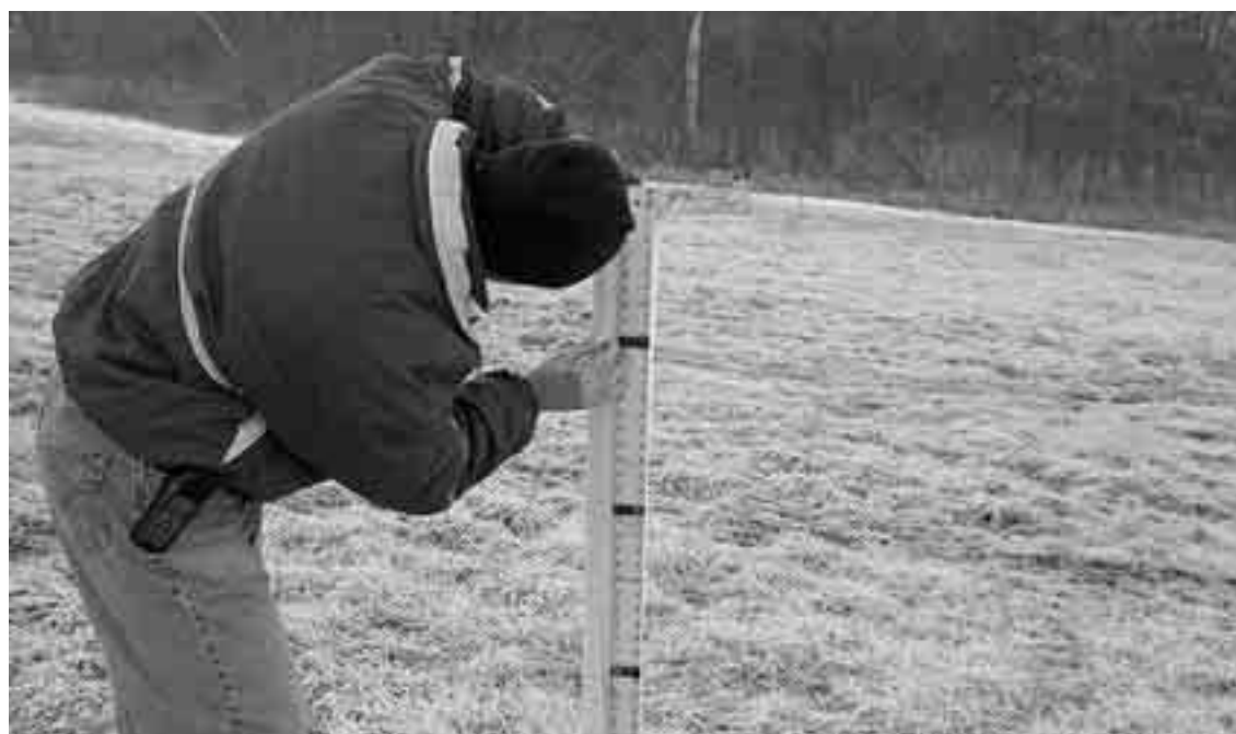
Photo 5-2. Person Marking a Post with a Sheetrock Square.
