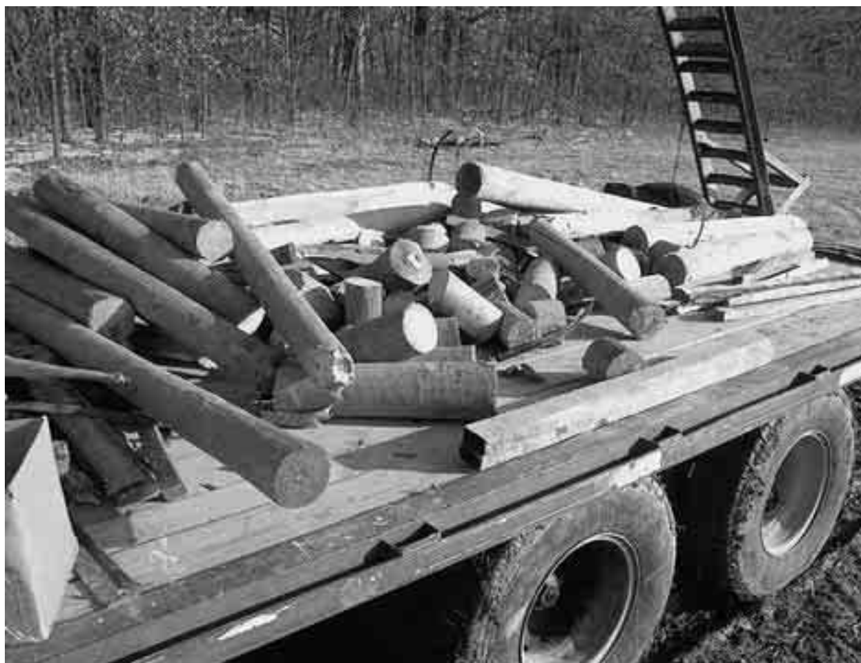
Photo 6-21. All of the debris from the installation needs to be picked up.
