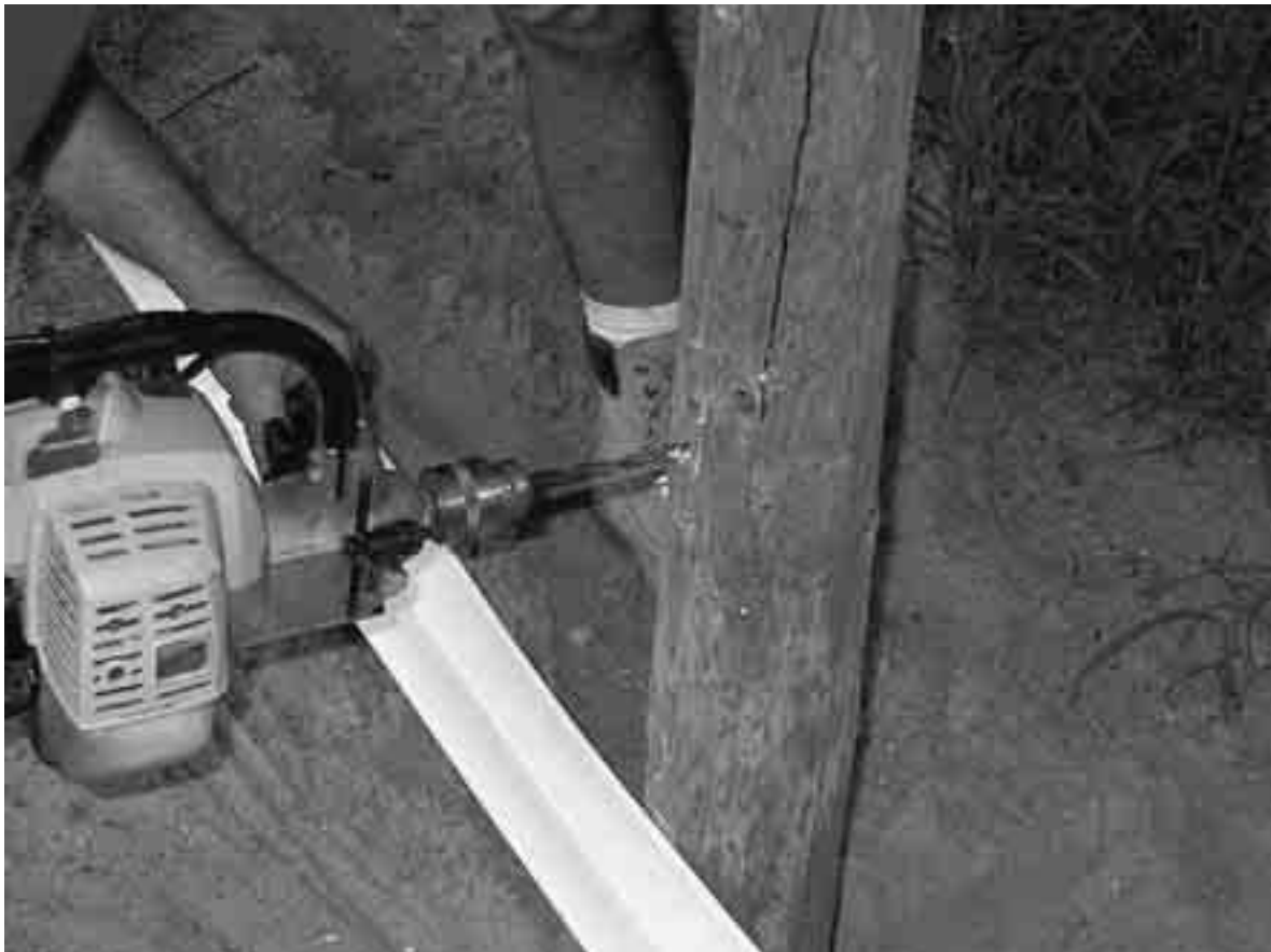
Photo A.1. Drilling a pilot hole using a 3/8" bit.
