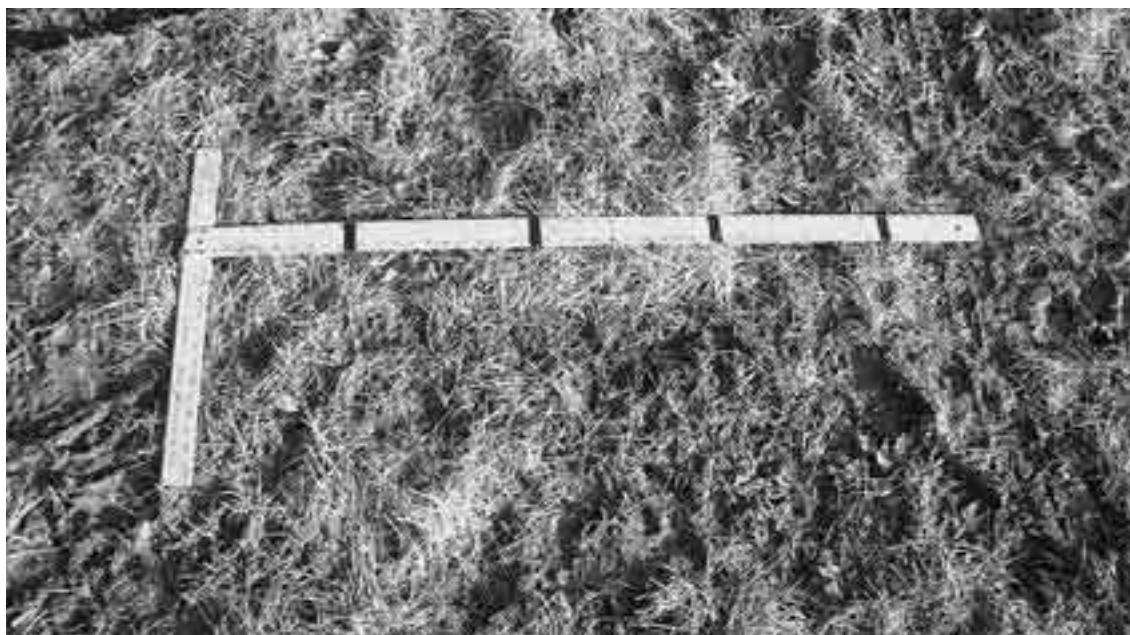
Photo 5-1. A sheetrock square ready to mark posts.
