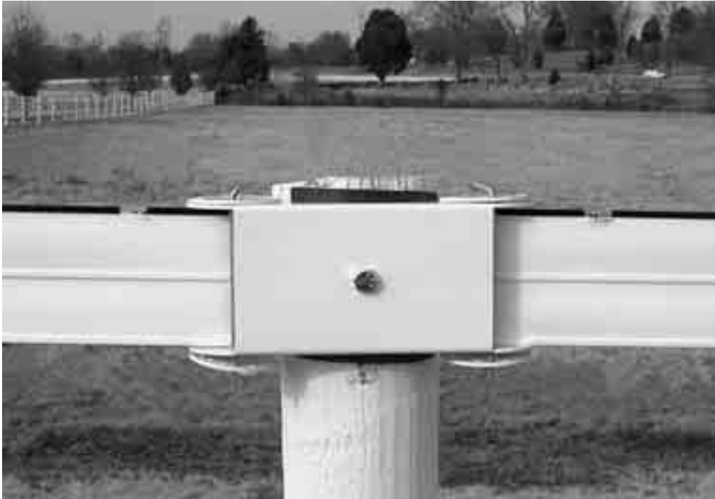
Photo A.8 A 2-way tensioner with connecting wire.
