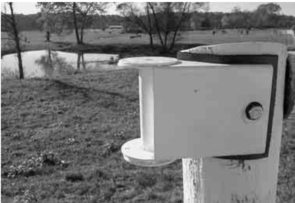
Photo A.3 A tensioner mounted on the post.
